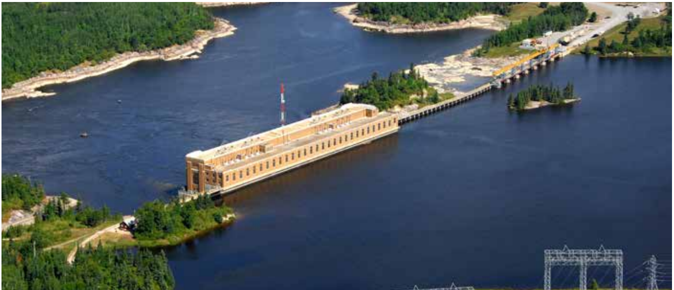
Slave Falls Generating Station is located on the Winnipeg River about 35 kilometres east of Lac du Bonnet.
