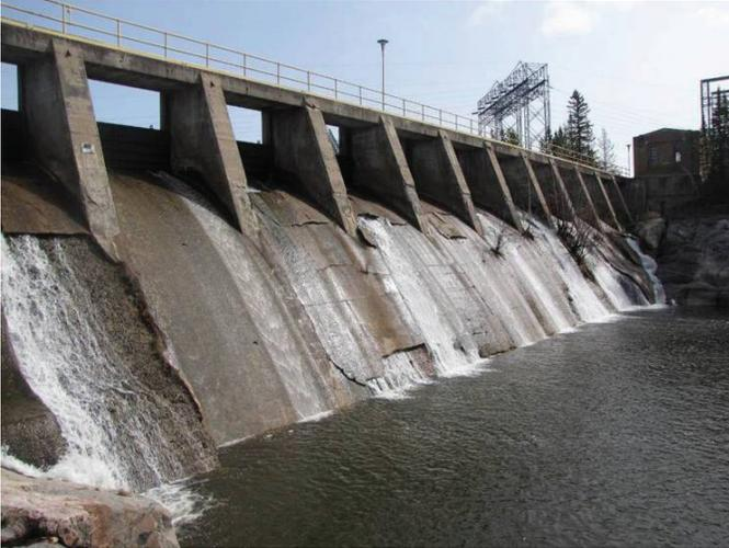
The Slave Falls Creek Spillway Project will reinforce the existing 85-year-old structure and convert it into a non-overflow dam. The Slave Falls Creek Spillway is located near the southern portion of the Slave Falls Generating Station.
